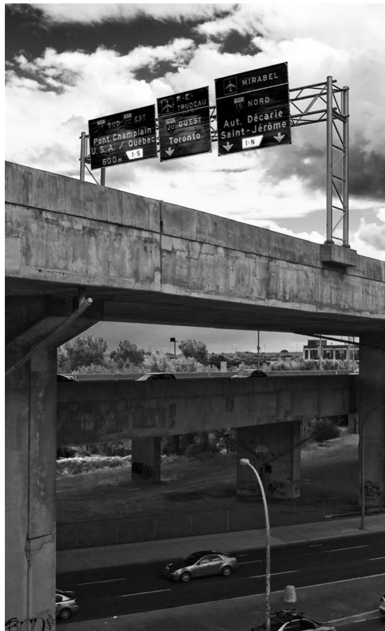
A view of the interchange from St-Henri. PHOTO JONATHAN DEMPSEY
