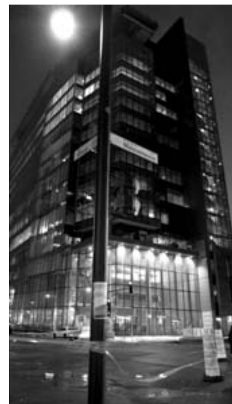
The streets around Concordia's still-unfinished JMSB building were closed on Dec. 28, 2008 due to falling glass from the structure. PHOTO JONATHAN DEMPSEY
