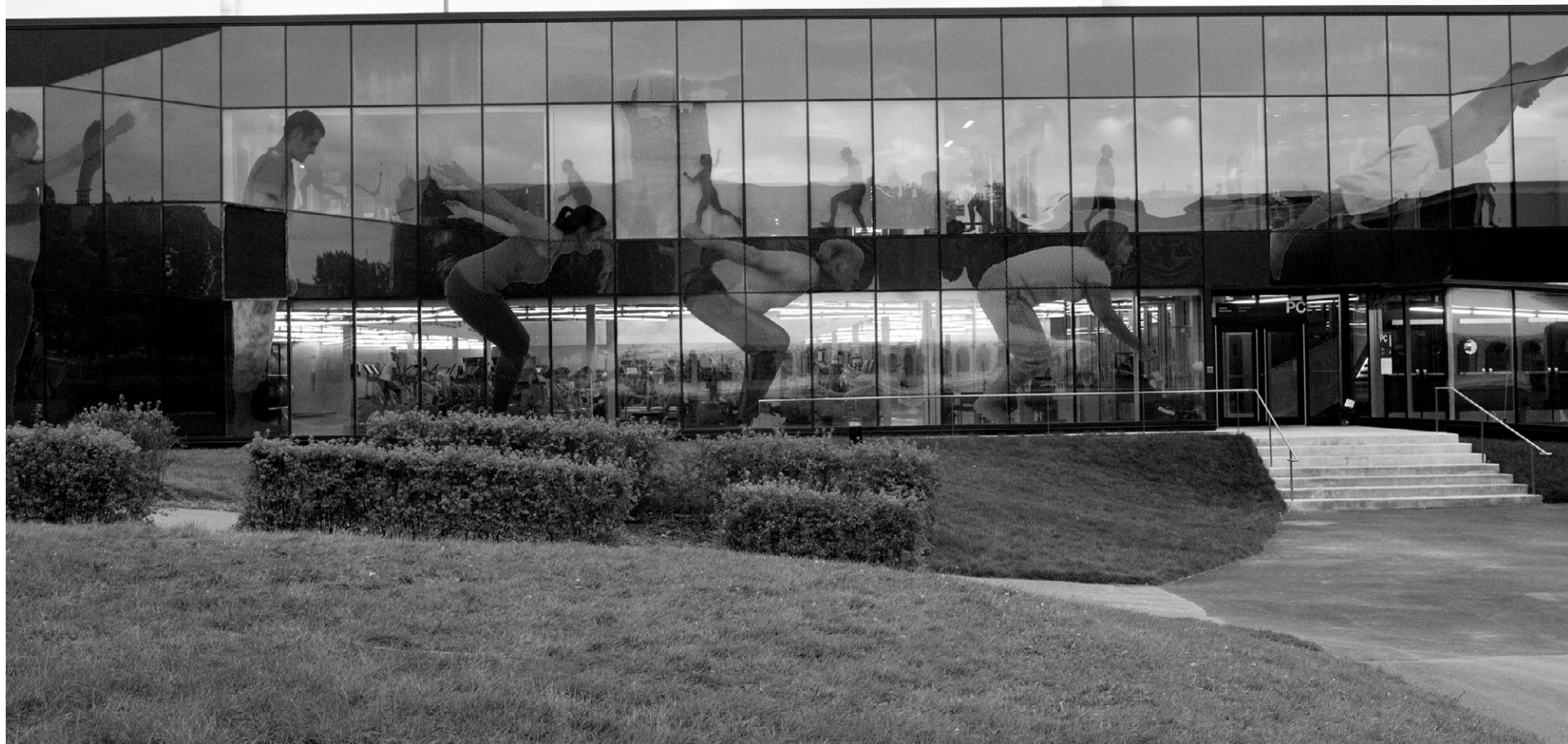
Concordia's new PERFORM Centre was built to meet the requirements of Leadership in Energy and Environmental Design.
